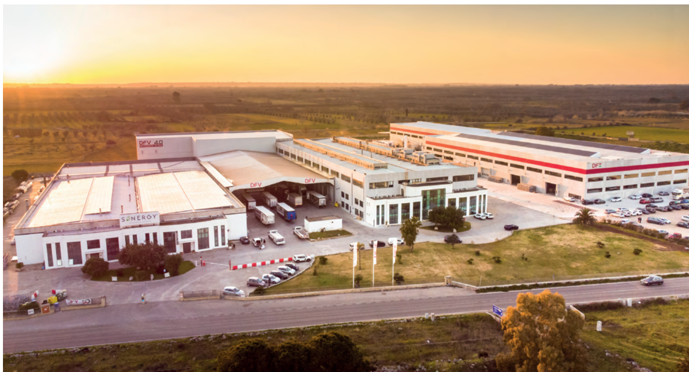
Surano (Lecce) - ITALY EXTRUSION - COATING - ARCHITECTURE
